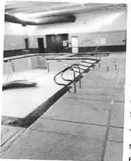
The center's pool liner was cracked, and the decking was beginning to chip. The cracking occurred when the center was closed during the pandemic in an effort to mitigate public health and safety concerns. The pool was closed and drained for both safety and cost saving measures, eliminating expenses for chemicals and heating the water. The liner cracked beyond repair during the closure, and the decking had already created safety concerns with loose surface rocks surrounding the pool and hot tub.
